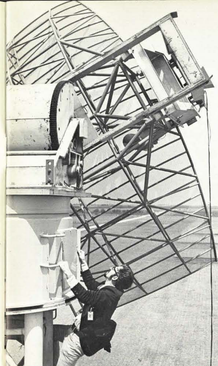
ASR-7 quality-assurance specialist Al Hockstein climbs testing tower to check some connections during final inspection of the radar antenna. Built in Dallas by Texas Instruments, the antenna is inspected at a test site outside the city.
