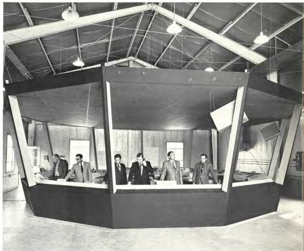
This mock-up is the exact size and shape of the tower cab to be placed atop the 180-foot-high shaft at the Dallas/Fort Worth Regional Airport. The tower with the 11-sided cab is scheduled to be completed next year.
