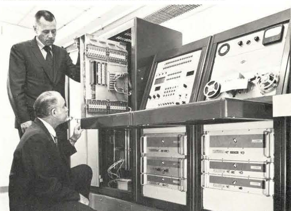
The two computers that make up Knoxville's conflict-detection system include the Univac 1230 with its magnetic-tape memory banks (left), being checked by Herbert Wachsman, FAA sub-program manager for the Systems Research and Development Service, and the Goodyear associative-array-processor computer (below), which works parallel to the Univac. Looking into the AAP are Wachsman and Russ Gall, Goodyear Aerospace Corp. engineer.—Goodyear photos
