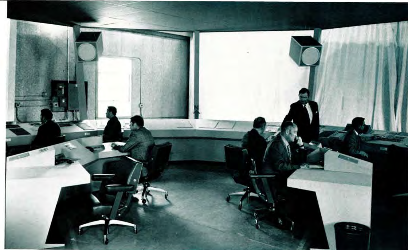
Southwest Region and NAFEC personnel man a full-scale mockup of the world's largest tower cab at Atlantic City where the new configuration is being tested. The 11-sided Undecagon-shaped, 620 square-foot cab will be the first of its type ever to be used by the agency. The 180-foot tower and cab is scheduled to go into operation April 1973 when the new Dallas-Fort Worth Regional Airport is opened. The tower will cost in excess of $2 million.
