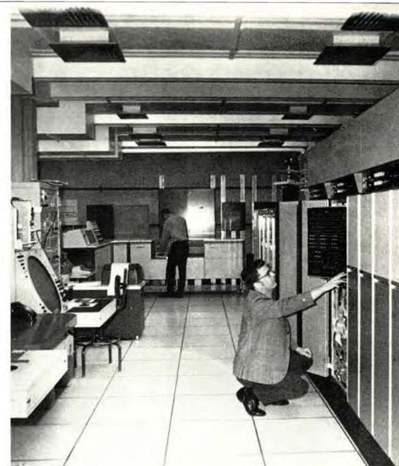
At Chicago-O'Hare, where the first operational ARTS-III has been installed, a computer processes information from aircraft and provides it to traffic controllers instantaneously. The data processing subsystem handles information which identifies the aircraft, its altitude and its speed.
