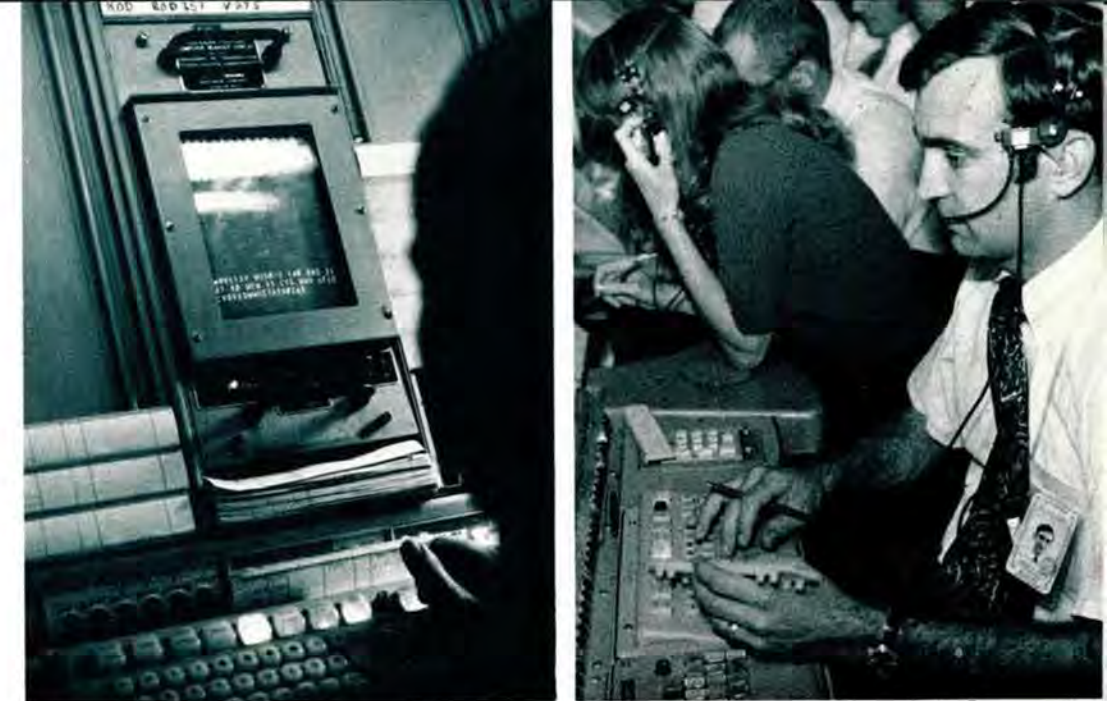
Computer message looks like this (left) to William D. Kinzie, controller at the Indianapolis Center, shown at the keyboard of the Computer Update Equipment console. If message shown on the screen is correct, it is entered into the computer merely by pushing a button.
