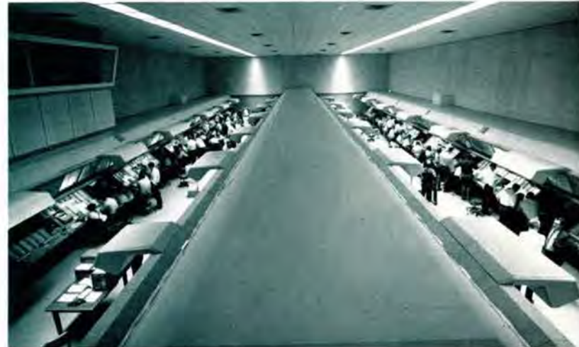
A clean sweep of uncluttered space in the new Cleveland Air Route Traffic Control Center stretches below the glass-enclosed visitors' balcony. Air ducting (center) draws hot air pockets away from the working positions. Similar ducting is tucked behind the consoles on either side.
