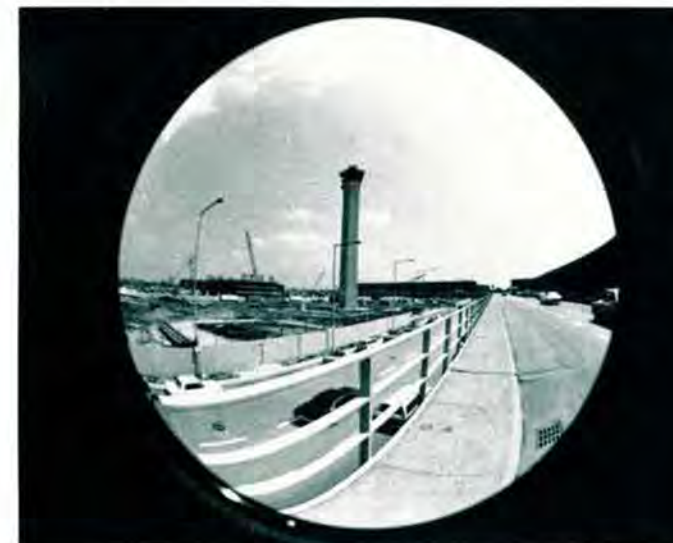
Stretching nearly 200 feet in the air, a new $5 million air traffic control tower has started handling traffic at O'Hare International, the world's busiest airport. The TRACON room, administrative offices, equipment room, computer complex and training facilities are all housed in 25,000 square feet below ground.
