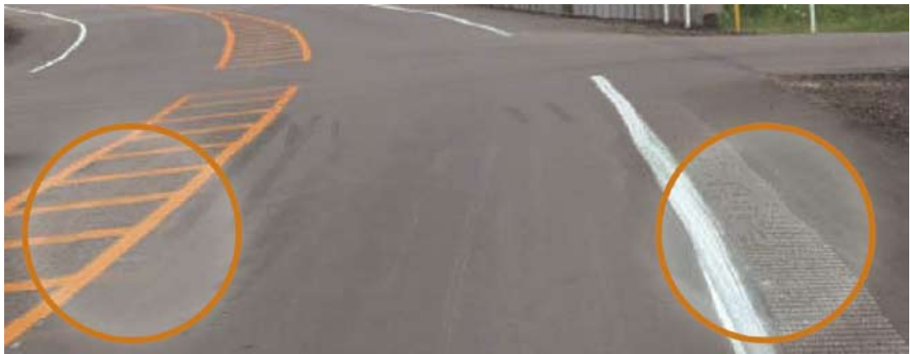
Figure 6: Lane Narrowing Using Rumble Strips
