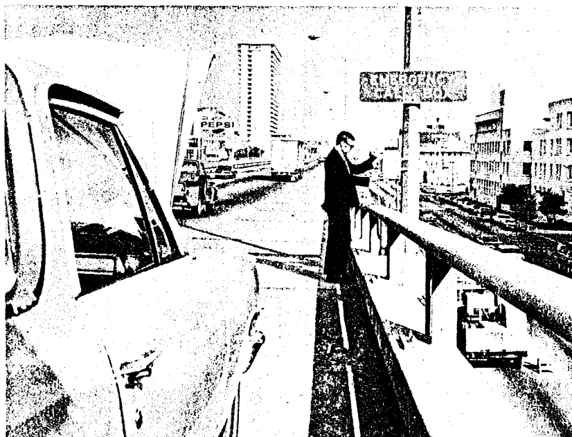
Figure 2. TYPICAL CALL BOX INSTALLATION.
