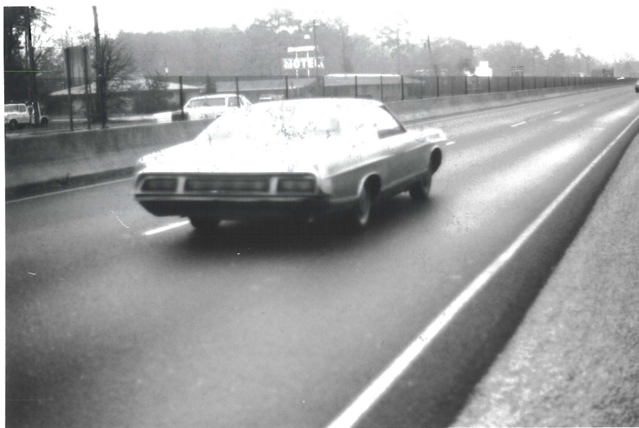
Figure 17. Splash and Spray Behind Automobile in 0.25 in/h Rainfall K_{avg} = 0.11 ; Location: 10/289/R 2/9/78
