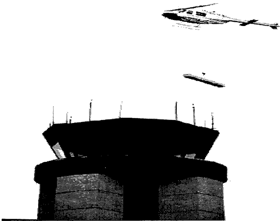
Figure 2-3. Helicopter Lift of Antenna and Pedestal.
