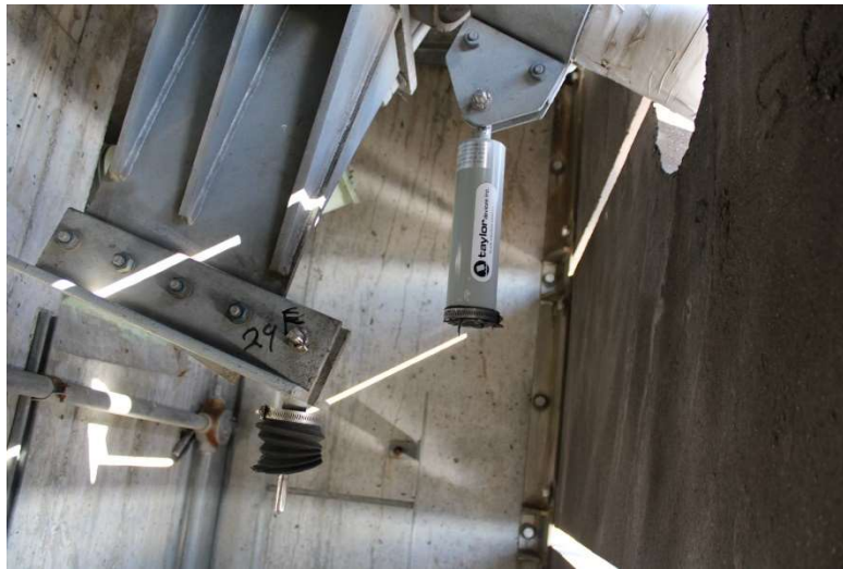
Figure 20 – Photo of Broken Damper at Cable E29
