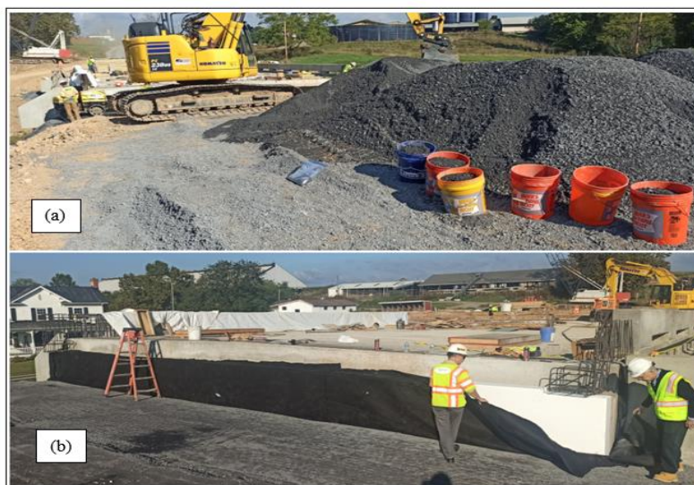
Figure 2. (a) Stockpile of Backfill Aggregate; (b) Installation of Expanded Polystyrene at the Bridge Construction Site over Route 682
