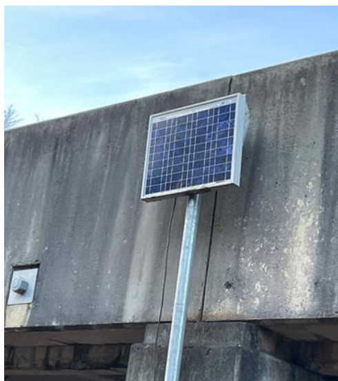
Figure 65. BIN 015002, Enterprise, AL. Solar panel powering the system.
