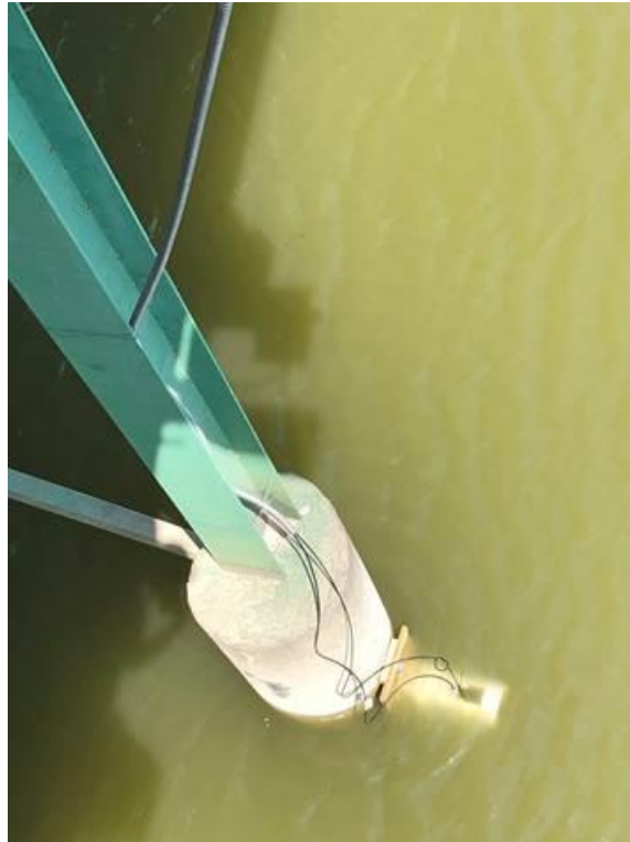
Figure 72. BIN 007070, Demopolis, AL. Installation on pier 4.
