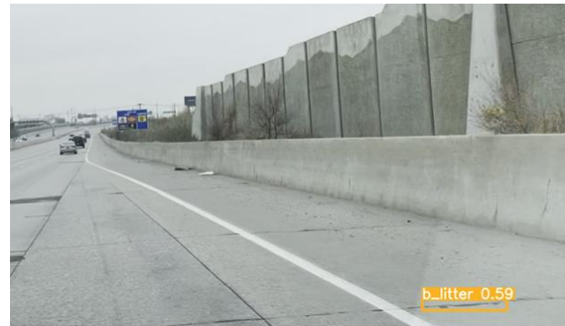
(b) Almost Fully Faded Marking
