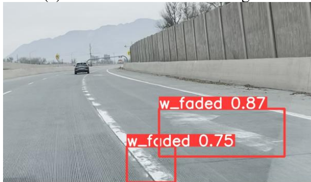
(e) Faded White Arrow and Lane Markings-1
