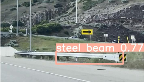
(a) W-Beam Steel Guardrail
