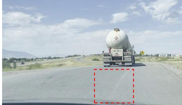
(b) Almost Fully Faded Marking
