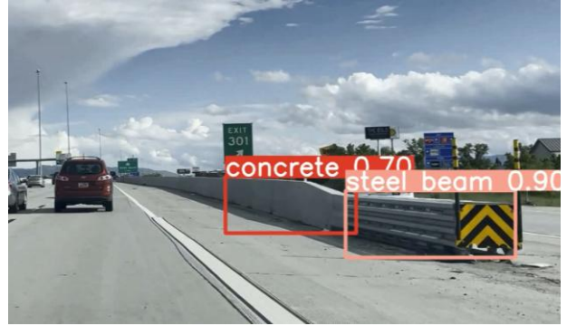
(b) Concrete Barrier and Steel Guardrail
