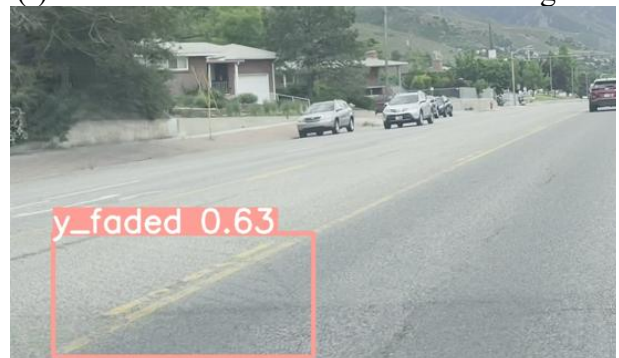
(h) Faded Yellow Double Lane Marking
