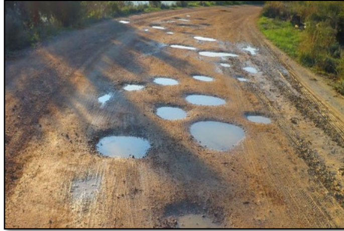
Figure 1.7 Formation of Potholes (KC Morgan, 2023)
