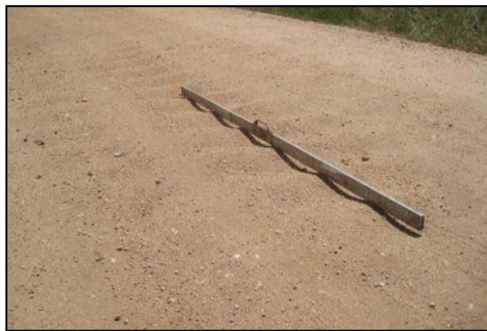
Figure 1.1 Poor riding quality due to washboarding (D. Jones, 2017)
