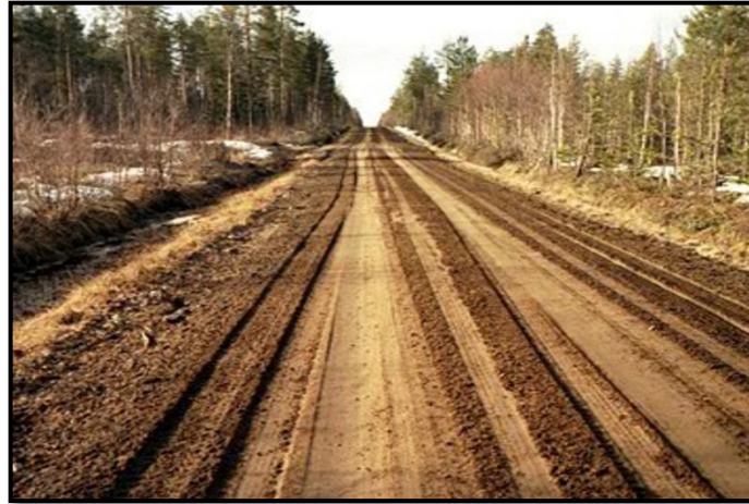
Figure 1.5 Severe rutting damage (ROADDEX, 2014)
