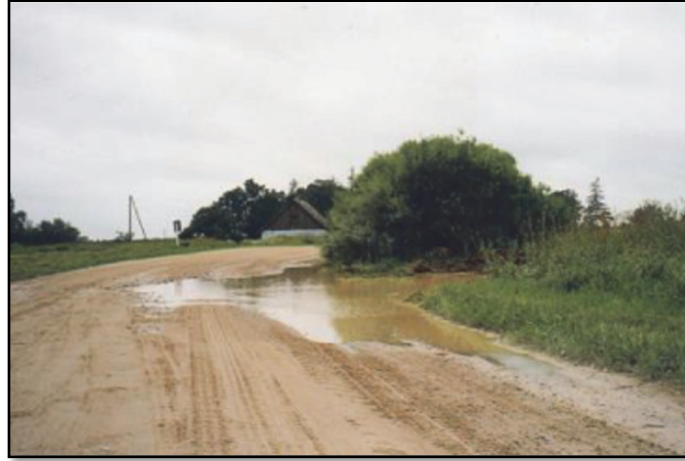
Figure 1.4 Impassible gravel road due to poor drainage (Saha & Ksaibati, 2017)
