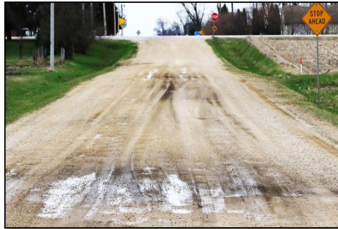
Figure 1.6 Seasonal damages due to freezing-thawing cycles (Jennifer DeWitt, 2019)
