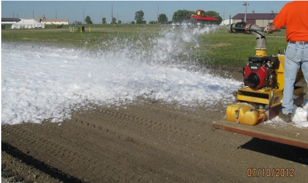
Figure 2.4 Straw blower used to distribute the fiber in the Iowa Expo project (White et al., 2013).
