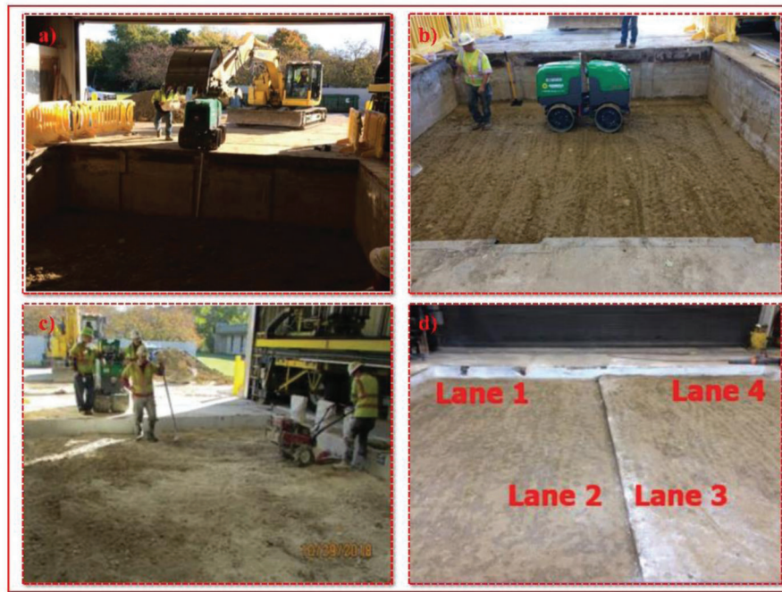
Figure 6.3 Construction of the subgrade layer.
