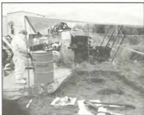
Bethel 1992, PCB spill; old electrical component put out in storage; less than 2 gallons of oil leak, 10 yards of soil removed
