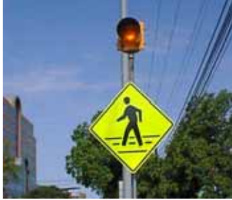
Figure 11-6. Photo. Flashing beacon treatment in Austin, TX.
