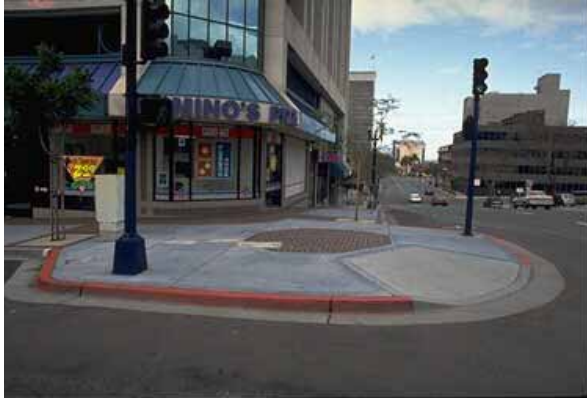
Figure 11-10. Photos. Curb extensions reduce crossing distances for pedestrians and provide additional corner storage space.
