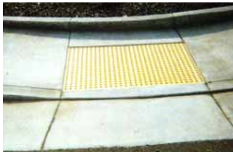
Figure 11-7. Photo. Detectable warnings treatment in Roseville, CA.
