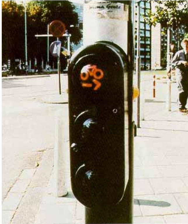
Figure 23-12. Photo. Bicycle signal used in Amsterdam, The Netherlands.
