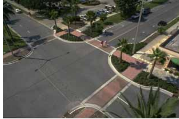
Figure 11-10. Photos. Curb extensions reduce crossing distances for pedestrians and provide additional corner storage space.
