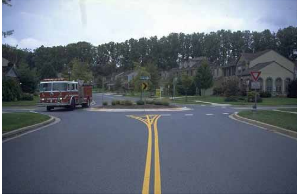
Figure 20-4. Photo. Emergency vehicle access should always be considered when incorporating traffic-calming measures.
