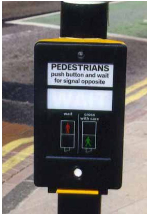
Figure 23-3. Photo. Pedestrian pushbutton for pelican signals in the United Kingdom.
