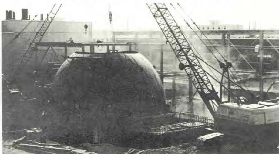
Cover for atomic reactor being built near Big Delta.
