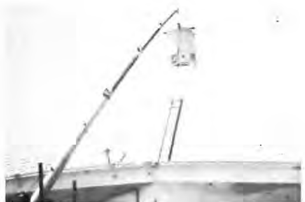
Nav Aids Section Chief, Leo J. Tabaka coordinates with crane operator as the antenna is lowered into final position. STL TACAN will soon be serving pilots on a 24 hour basis.
