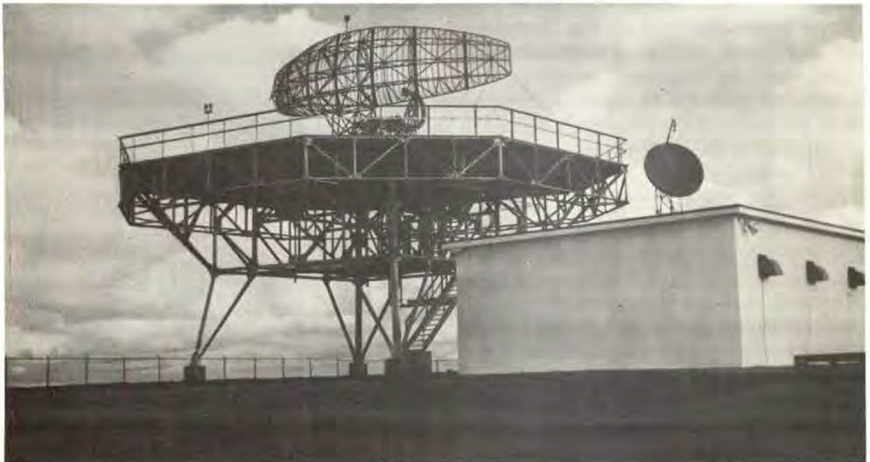
ARSR facility which takes the picture to be transmitted by the RML to the ARTCC.
