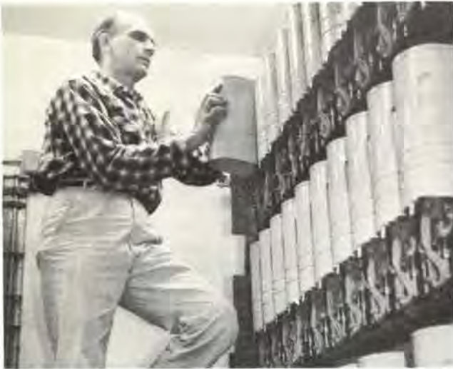
Gene Doran (Southwestern Bell Telephone employee) adjusts switch-board equipment. The can he holds is called a line finder and locates a vacant line for you when you dial Nine.
