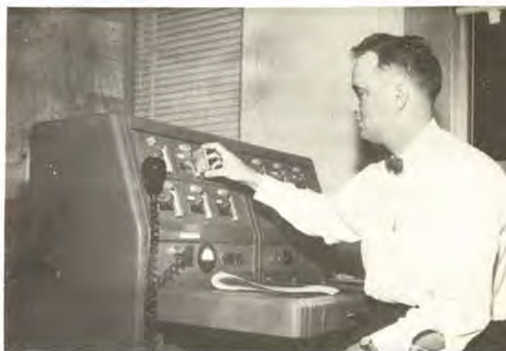
Robert B. Dalton, Jr., Airways Operations Specialist at the Wichita FSS, inserting a cartridge of fresh weather information in the Transcribed Weather Broadcast Unit there.
