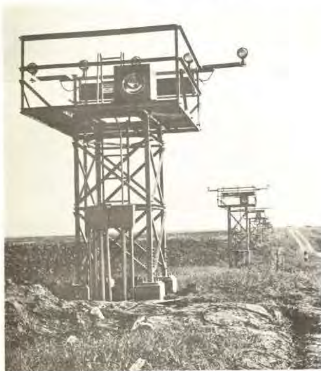
A 5-light center line bar with sequenced flashing lights showing the type support presently used for all lights requiring a structure from 11'6" to 124' in height. View shows the one at Capitol Airport, Springfield, Illinois.
