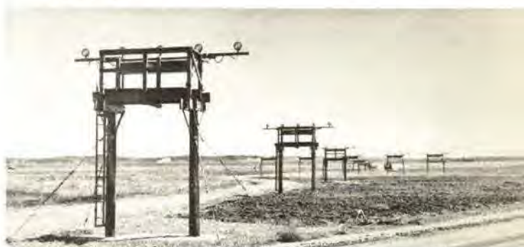
View of a 5-light center line bar used at Municipal Airport, also at Omaha. In the background is the 1000-foot distance marker bar.
