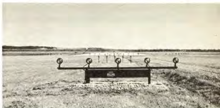
Photo shows a 5-light center line bar which is used when light supports are less than 6 feet in height - Municipal Airport, Omaha, Nebraska.
