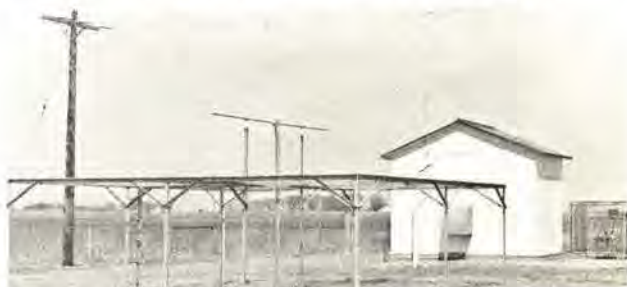
The Middle Marker, which provides a positive check point on the landing approach.
