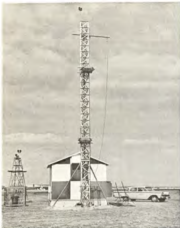
Glide Slope Site featuring new type antenna mast. At left is Weather Bureau Transmissometer.
