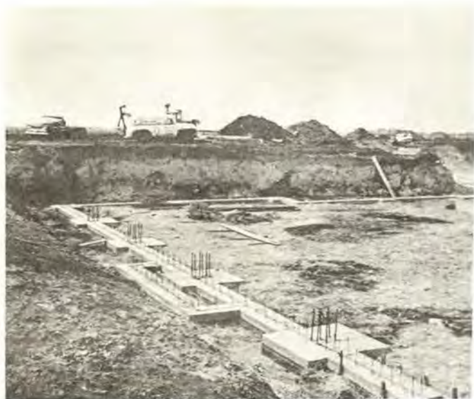
After fighting a battle of winter mud, foundations are poured for the new Chicago ARTCC.
