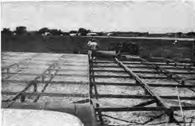
Horizontal counterpoise screen under construction at the Des Moines glide slope.
