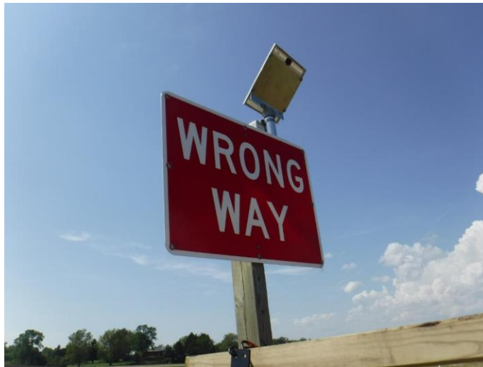
Figure C.20: Installation of Flashing LED Wrong Way Sign at Auburn Rd Ramp
