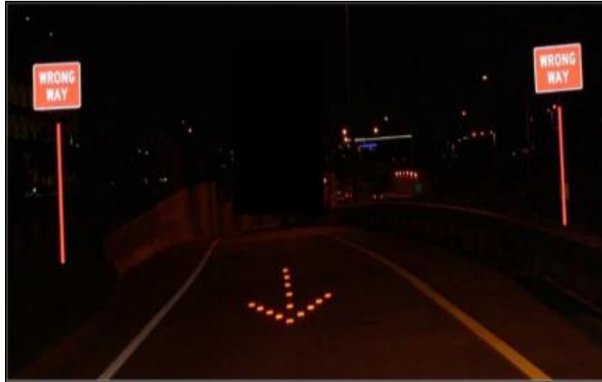
Figure 2.4: Wrong-Way Arrow with RRPMs and Supplemental Wrong-Way Signs Source: Zhou & Pour-Rouholamin (2014)
