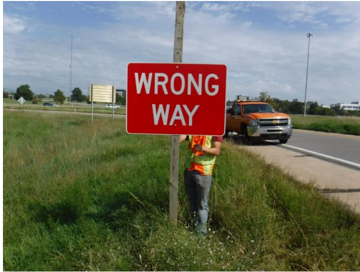
Figure C.19: Installation of 2nd Oversized and Lowered Wrong Way Sign on Wanamaker South Ramp
