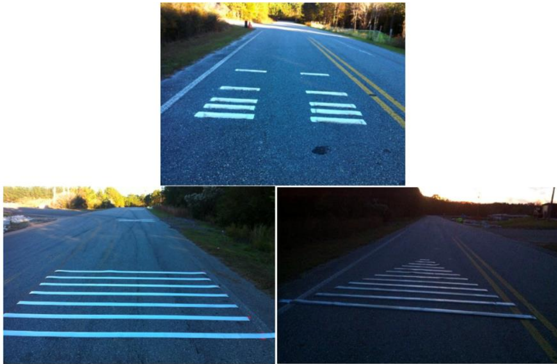
Figure 2.3: Effective Directional Rumble Strips
