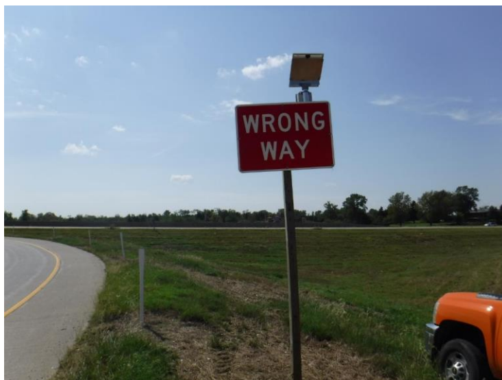
Figure C.21: Installation of Flashing LED Wrong Way Sign at Auburn Rd Ramp
