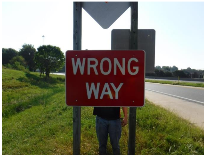
Figure C.16: Installation of 2nd Oversized and Lowered Wrong Way Sign on Wanamaker Rd North
