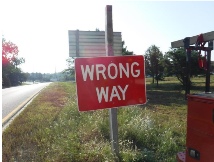
Figure C.14: Installation of Oversized and Lowered Wrong Way Sign at Gage Blvd Ramp
