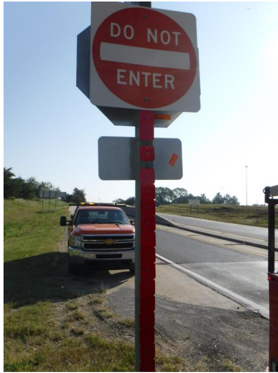
Figure C.15: Installation of RRFDs on Gage Blvd
