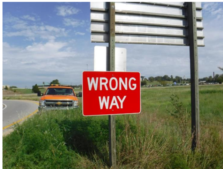
Figure C.18: Installation of 1st Oversized and Lowered Sign at Wanamaker Rd South Ramp
