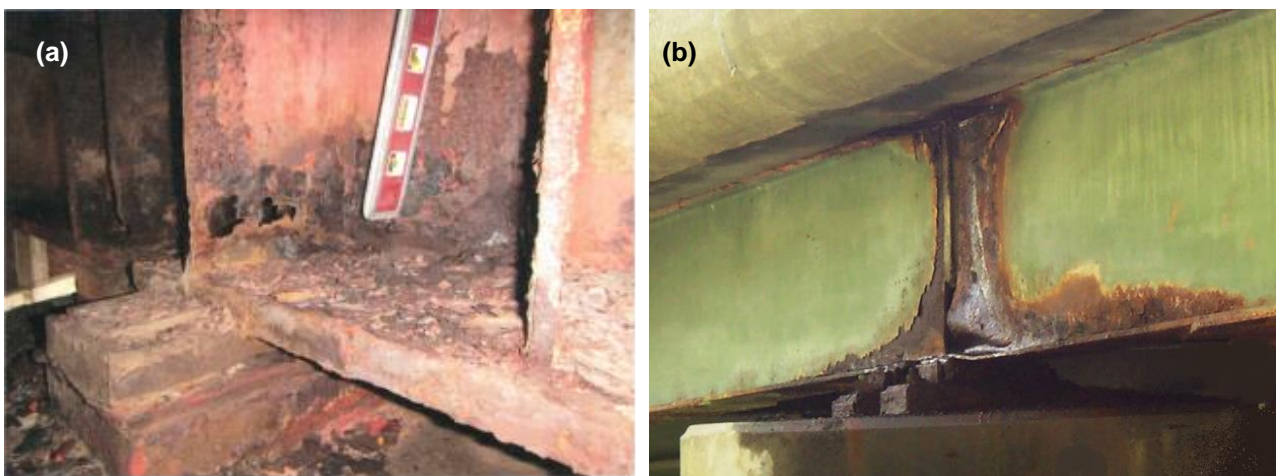
Figure 1. Corrosion at beam end resulting in (a) a hole in the bearing stiffener (Photo Courtesy of Luis Vila) and, (b) web crippling (Photo Courtesy of Michael Culmo).
