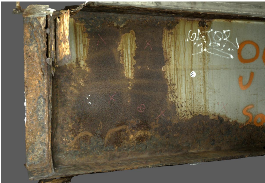
Figure 2. Sample of 3D model of corroded bridge beam generated with 3D scanning.
