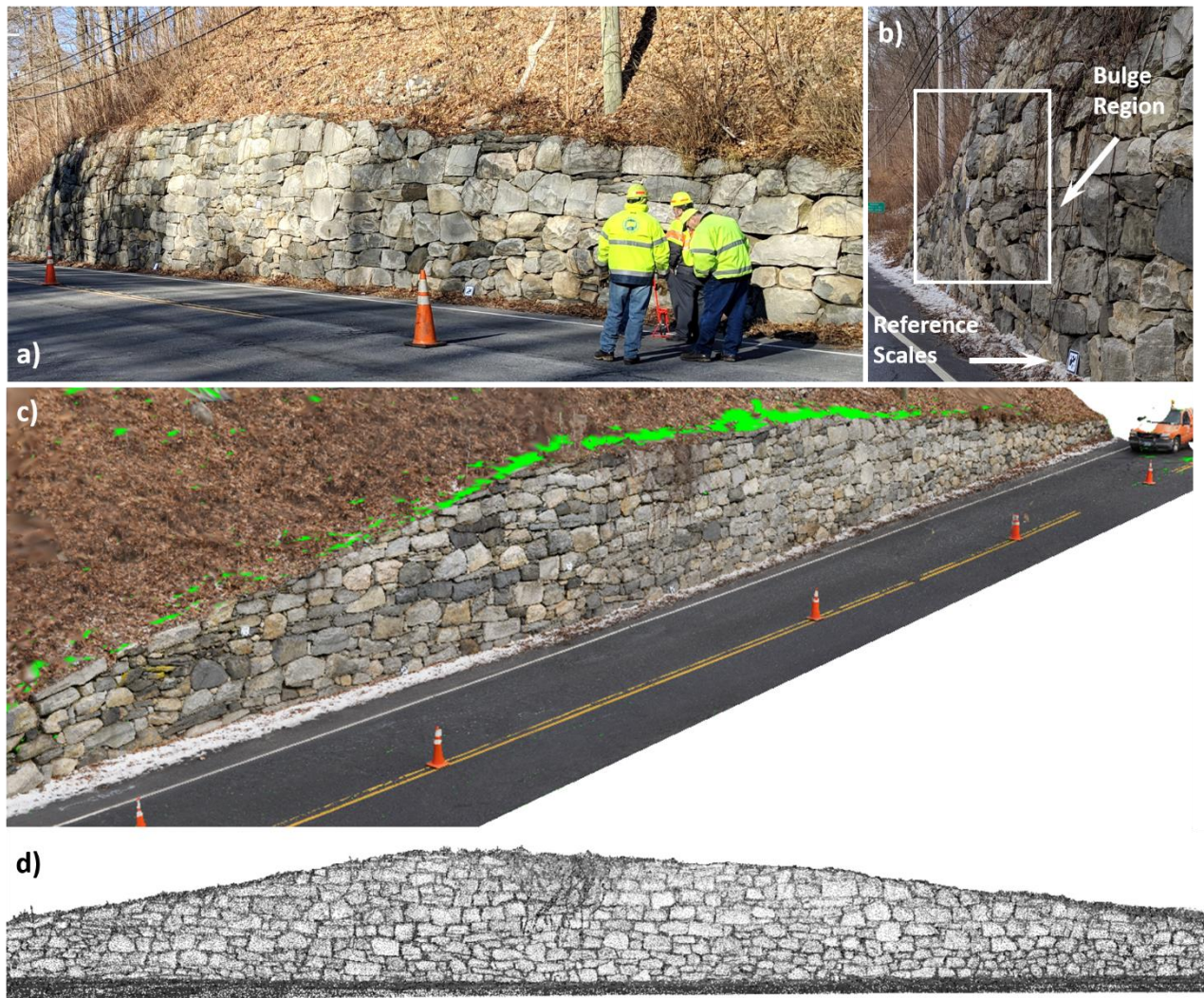
Figure 2. Retaining wall from Field Trial 1 in Connecticut showing a) overall view of wall, b) closeup of bulge region, c) image of 3D model of wall, and d) point cloud.
