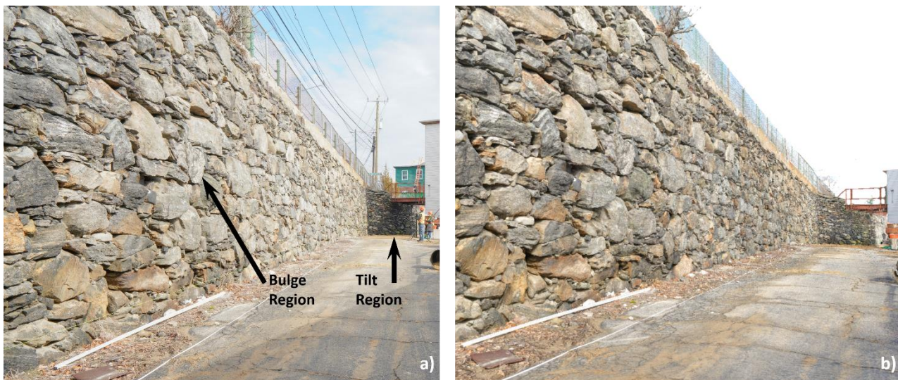
Figure 3. Retaining wall from Field Trial 2 in Connecticut showing a) picture from site and b) snip of 3D model.
