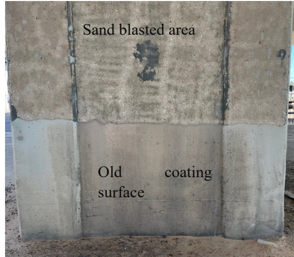
Surface before and after sandblasting
