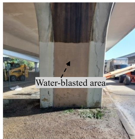
Surface before and after water-blasting
