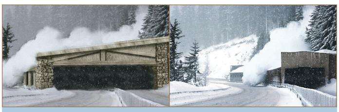
This design visualization shows a new snowshed (left), slated for construction in 2011, with an avalanche tumbling over it. The structure covers the lanes in both directions, helping protect motorists traveling through Snoqualmie Pass from experiencing the brunt of an avalanche. The original snowshed (right) protected only the travel lanes closest to the mountainside.
