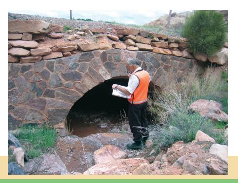
The WIP accounts for both primary and secondary wall types. Here, at Colorado National Monument, an inspector assesses a mortared stone masonry culvert headwall topped by a secondary dry-laid stone wall.
