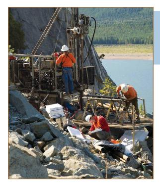
WSDOT and contractor crews drill and log core samples along a cliff in the project area to obtain information on the slope's stability.
