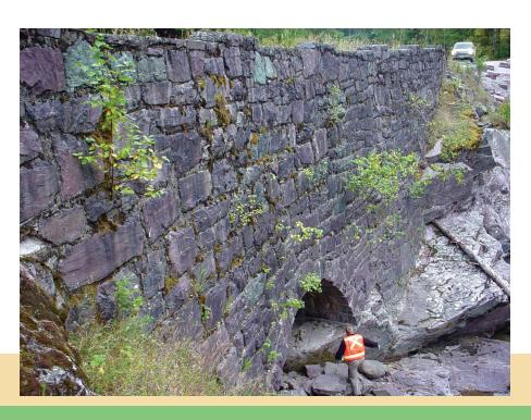
Retaining walls associated with bridges may or may not qualify for the WIP inventory. FLH inspectors determined that this dry-laid stone masonry wall in Acadia National Park supports the bridge approach and should be included in the WIP survey. The mortared stone masonry wall along the bridge abutment, however, would be assessed under the Bridge Inspection Program.
