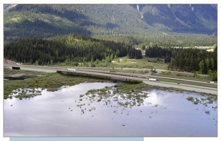
This design visualization shows the new Gold Creek Bridges, which will allow wildlife to cross safely under the interstate and will improve stream channel migration and fish passage. Fences will guide wildlife safely under the bridges.
