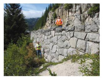
At Mount Rainier, a team surveys a mortared stone masonry wall. One person measures wall dimensions while the other records element conditions.
