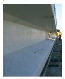
University of Minnesota researchers found that prestressed concrete girders cast with self-consolidating concrete and no vibration (shown here) require fewer surface repairs than those cast with conventional concrete and internal vibration. Photo: Bulent Erkmen.
