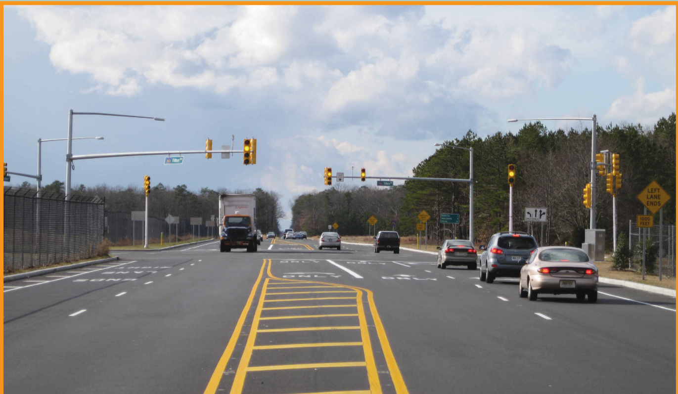
Atlantic County, NJ, used CRFs to select a combination of safety improvements to reduce right-angle and same-direction crashes at the intersection (above) of Tilton Road (County Route 563) and Wrangleboro Road (County Route 575). The reconstructed intersection (below) includes left-turn lanes on all four approaches, bike lanes, and signal timing modifications. Photo: John A. Masi, Atlantic County, NJ, Division of Engineering, Department of Regional Planning & Development.
