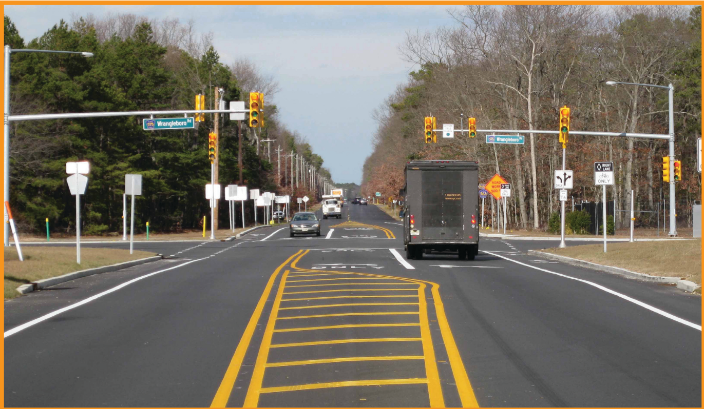
Atlantic County, NJ, used CRFs to select a combination of safety improvements to reduce right-angle and same-direction crashes at the intersection (above) of Tilton Road (County Route 563) and Wrangleboro Road (County Route 575). The reconstructed intersection (below) includes left-turn lanes on all four approaches, bike lanes, and signal timing modifications. Photo: John A. Masi, Atlantic County, NJ, Division of Engineering, Department of Regional Planning & Development.
