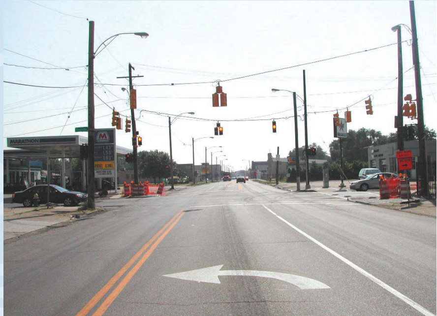
These before (left) and after (right) photos depict the intersection of 7 Mile Road and Dequindre Road in Detroit, MI. An RSA in 2002 led to, among other changes, placement of a left-turn arrow on the pavement to improve roadway navigation and safety. Photos: AAA Michigan.
