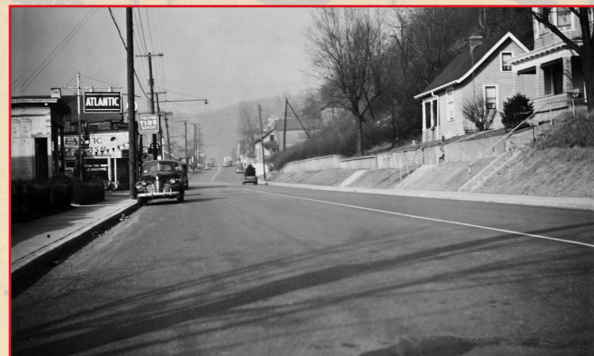
This section of the National Road (U.S. 40) in Wheeling, WV, was reconstructed in 1941 to provide a road width of 12 meters (40 feet).
