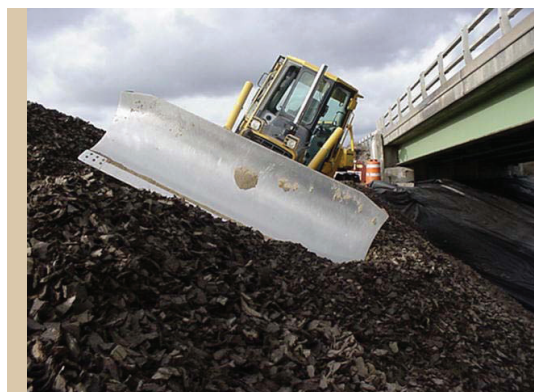
A bulldozer is leveling a pile of shredded tires that are being reused as lightweight fill for a bridge abutment and slope. Recycling is one aspect of creating greener highways.
