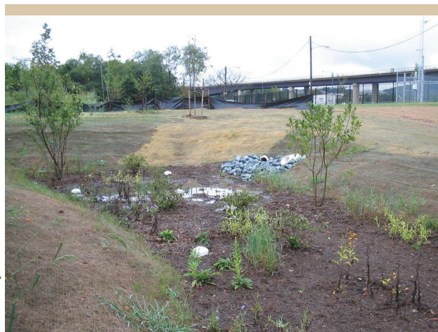
This lowland area is a bioretention facility on Benning Road in Washington, DC, designed to manage stormwater.
