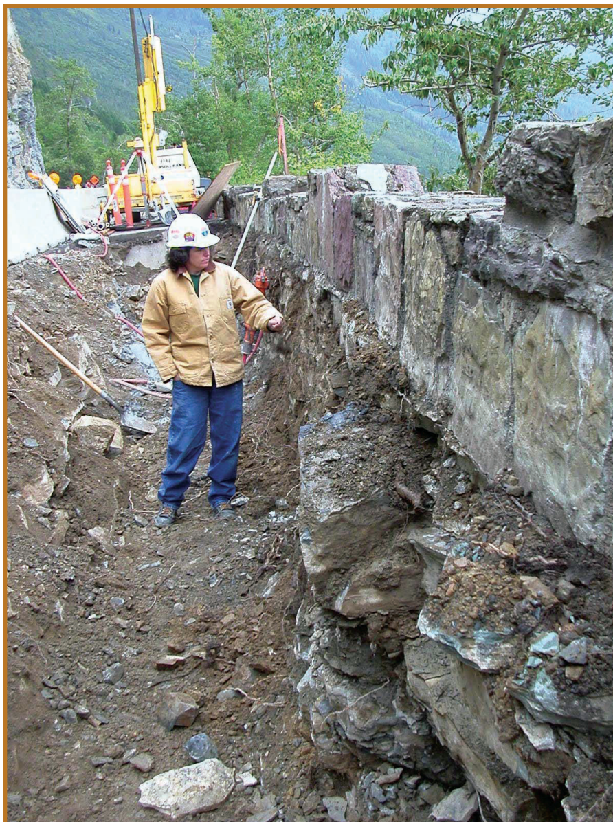
FHWA Resident Engineer Margaret Moen, who worked on the project until early 2006, inspects a construction site where a new and hidden concrete retaining wall was constructed inside the original wall, allowing the historic wall to maintain its original appearance without having to support its former structural load.
