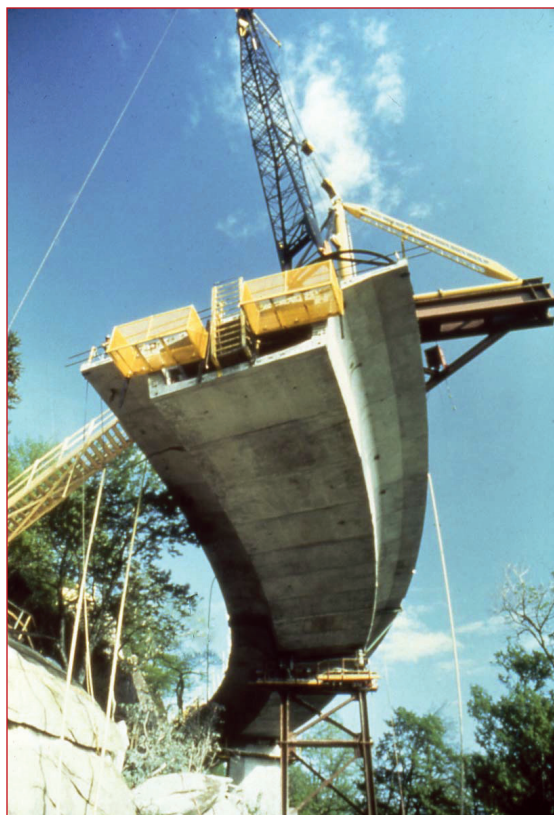
Building the Linn Cove Viaduct from the top down obviated a significant footprint on ecologically rich Grandfather Mountain in North Carolina.
