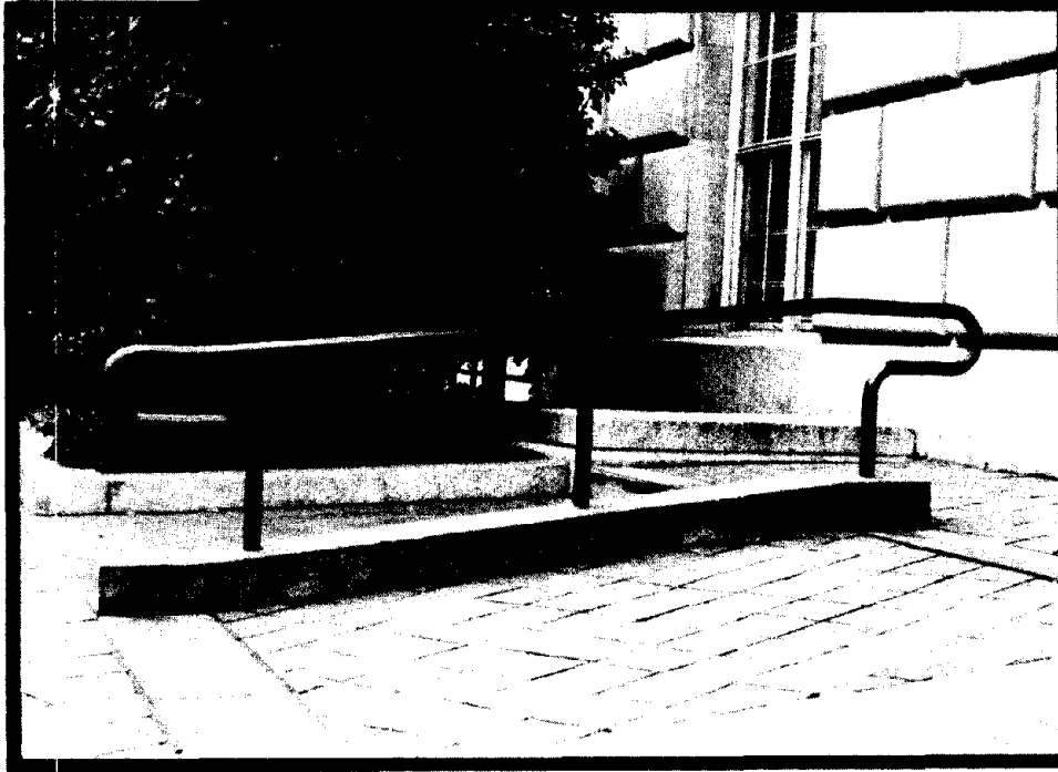
Figure 69. Handrail end extension.
