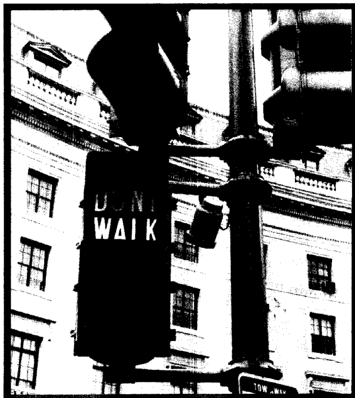
Figure 89. Audible pedestrian signal.
