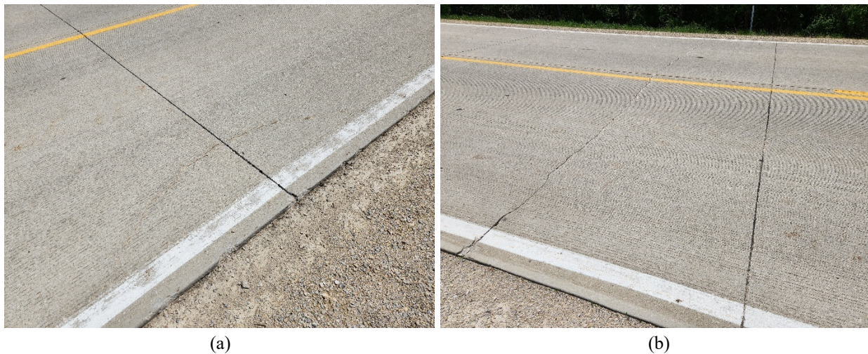
Figure 32. Typical (a) corner and (b) transverse cracking observed at Site 4
