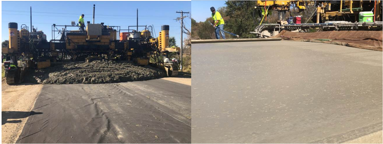
Figure 112. Construction photos from joint-free FRC overlay test section
