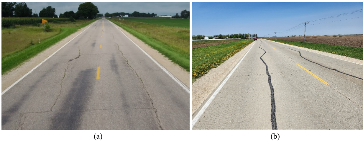
Figure 34. Longitudinal cracking at Site 4 (a) prior to overlay and (b) post-overlay
