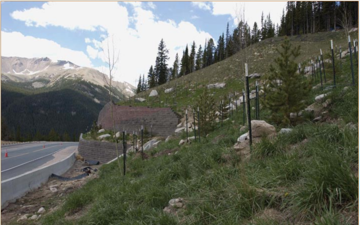
The terraced and revegetated slopes shown here along mountainous U.S. Route 40 in Colorado help reduce erosion and protect streams and the local watershed from sedimentation.
