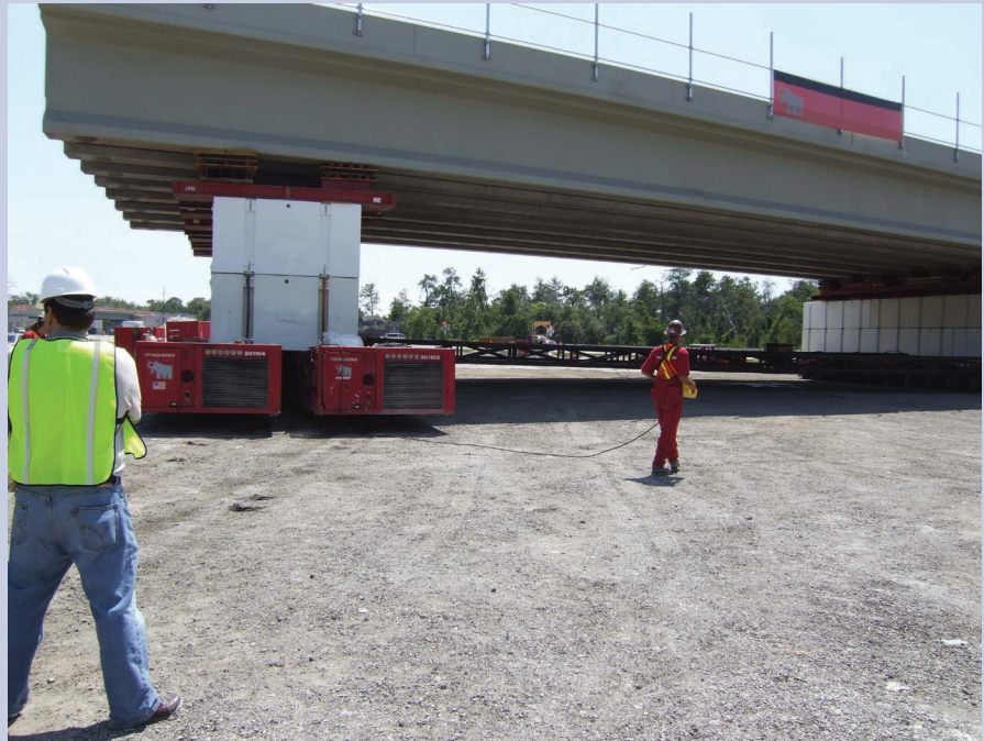
FDOT workers here use an SPMT to replace the span of the Graves Avenue bridge. FHWA will help promote such vanguard technologies through additional demonstrations.
