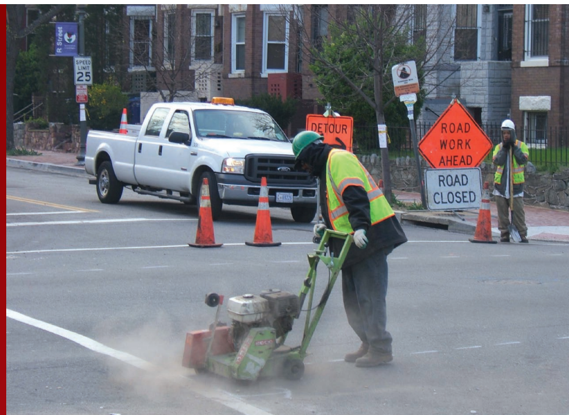
Another goal is the safety of construction workers, such as this man cutting through pavement at a residential intersection. Photo: Tim Breen for FHWA.
