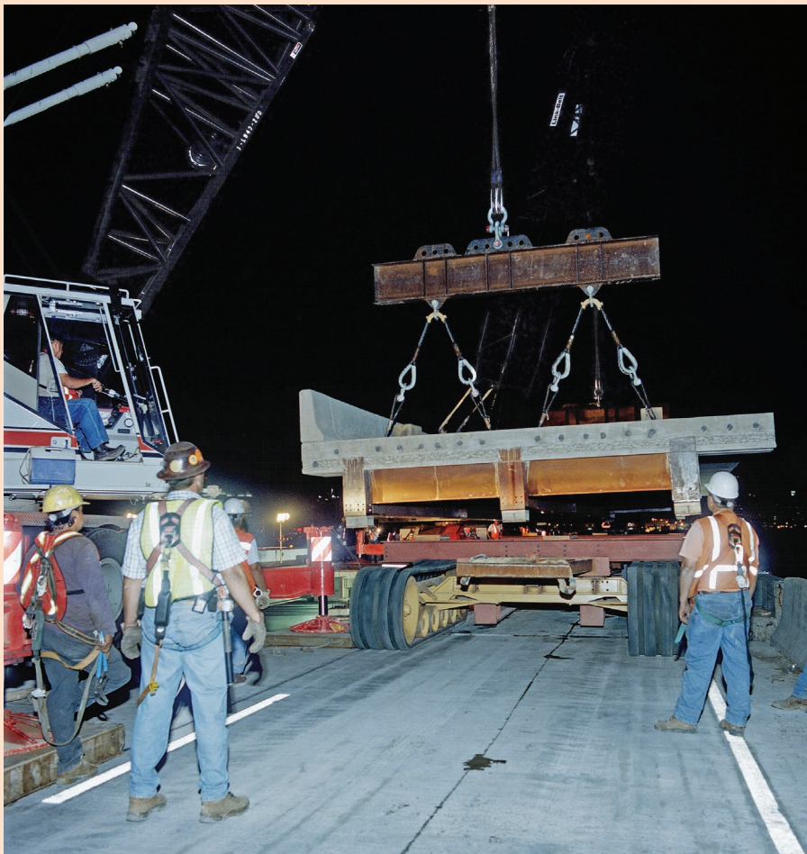
Prefabricated Bridge Elements and Systems (PFBES) were used on this I-95 project in Richmond, VA, to complete a bridge deck replacement. PFBES, an FHWA-supported priority, market-ready technology, allowed construction to proceed with only nighttime lane closures, saving the Virginia Department of Transportation (VDOT) an estimated 12 to 14 months of construction time. Photo: VDOT.
