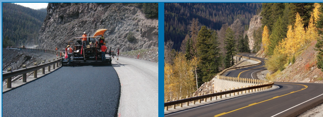
(Left) A work crew is using WMA to pave this section of the East Entrance Road inside Yellowstone National Park, WY, between the East Entrance Gate and Sylvan Pass in fall 2007. (Right) The completed road. Photos: Brad Neitzke, Western Federal Lands Highway Division.
