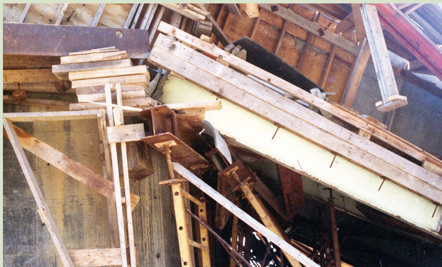
Shown here is a closeup of the northeast tower of the collapsed deck of Bridge No. 4. The screw jacks atop the shoring tower that hold the metal transverse cross-beams appear to be slightly bent. The hardwood blocking used to increase the deck elevation is above and to the left of the screw jacks.
