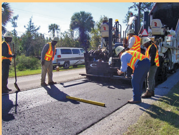
A crew in Deland, FL, checks to ensure a high-RAP pavement is level.
