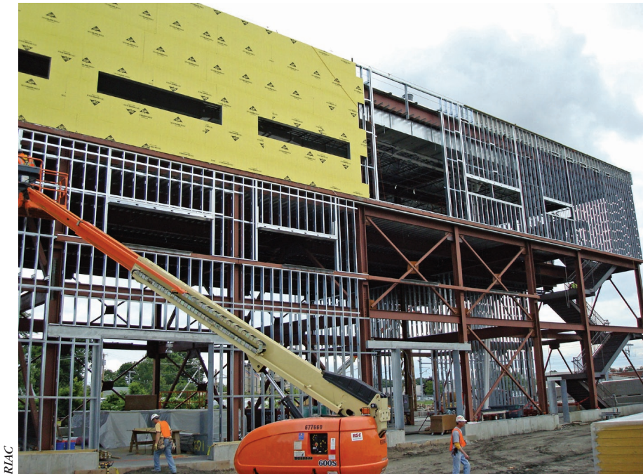
Installation of paneling and sheathing is shown at the building that will house rental car counters and offices.
