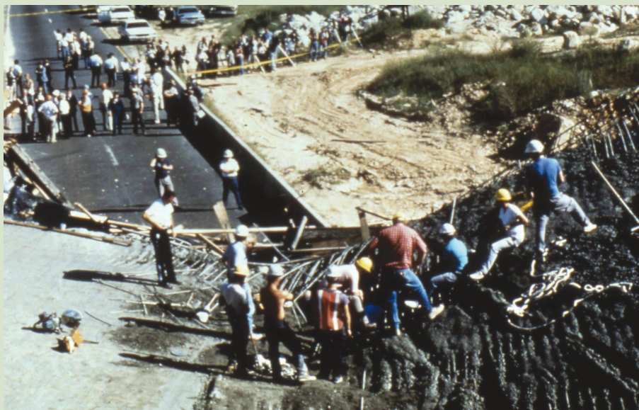
Workers are dismantling the collapsed bridge elements from Bridge No. 4. Shot from Bridge No. 2, this photo shows a portion of the bridge surface with set concrete (left) and the point of collapse, with the rebar part of the section that collapsed (right).
