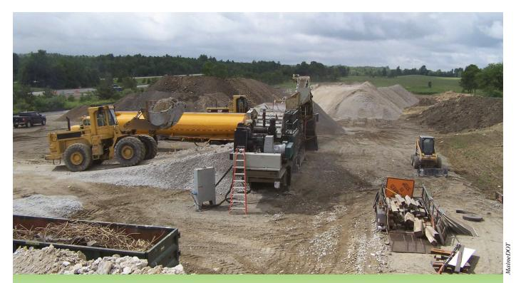
The contractor established this onsite recycling and staging area where a portable crusher (shown here) processed the waste concrete into shoulder aggregate.
