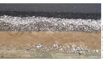
MaineDOT's use of a multilayered porous paving system (shown here) will help protect Long Creek Watershed from direct runoff from a heavily traveled roadway.
