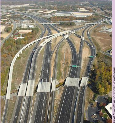
The system of collector-distributor roads shown here at the recently reconstructed I-85/SR-316 interchange northeast of Atlanta, GA, are auxiliary lanes separated from the freeway mainline to avoid conflicts between through traffic and local entering and exiting vehicles.
