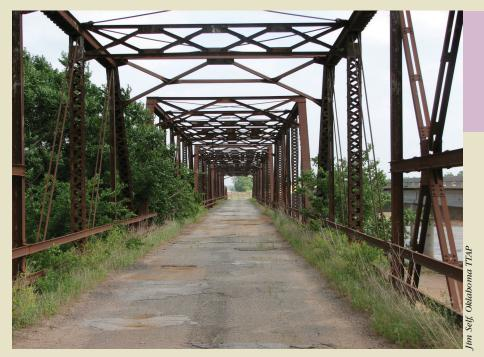
The old Cimarron River Bridge, a multitruss steel structure built circa 1927 in Kingfisher County, OK, now is closed to vehicle traffic because it is structurally unsound and unable to handle modern traffic loads and volumes.
