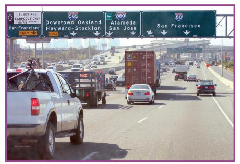
Overhead guide signs such as this multipaneled truss sign at the MacArthur Maze interchange in Oakland, CA, need to make the optional lane clear. A driver traveling in the far right lane might have difficulty discerning the interior optional lanes.
