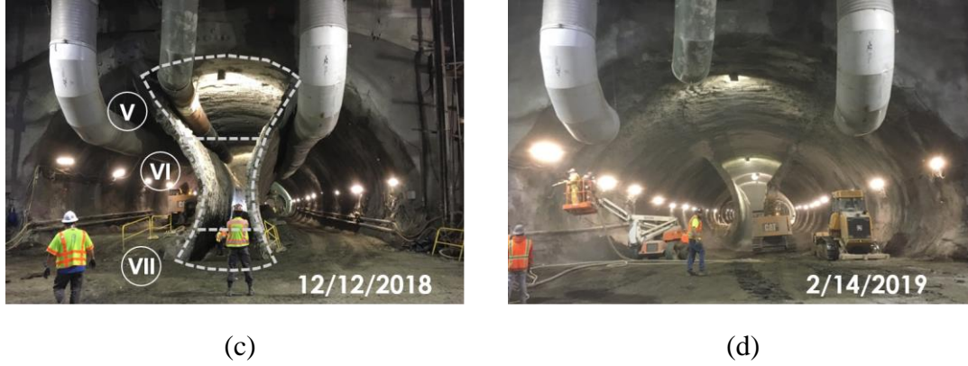
Figure 3.3 SEM construction progress: (a) Left drift (I: left top heading, II: left invert); (b) Right drift (III: right top heading, IV: right invert); (c) Center drift (V: center top heading, VI: center bench, VII: center invert); and (d) Temporary wall demolition.
