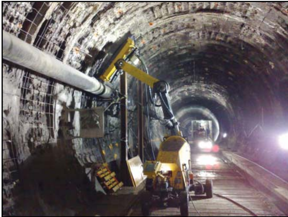
Figure 2-9: Hydroexcavation robot removing damaged concrete in tunnel liner [7].
