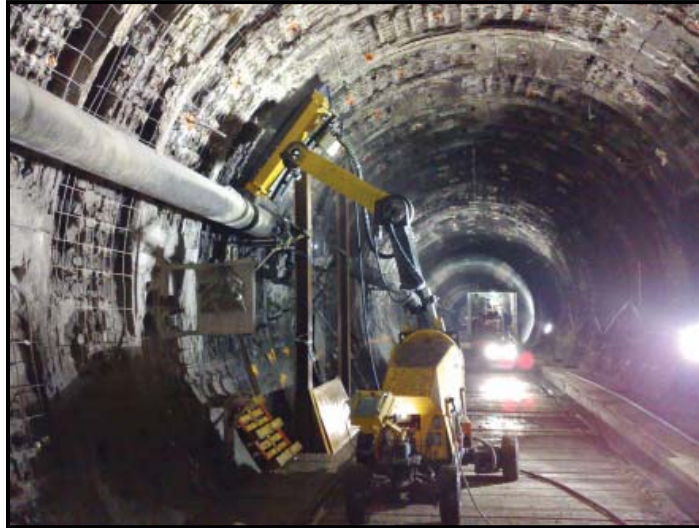
Figure 1-2: Hydroexcavation robot removing damaged concrete in Channel Tunnel liner [7].
