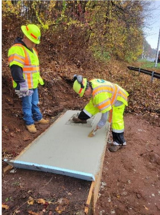
Figure 2.9. Concrete Slab Brush Finish
