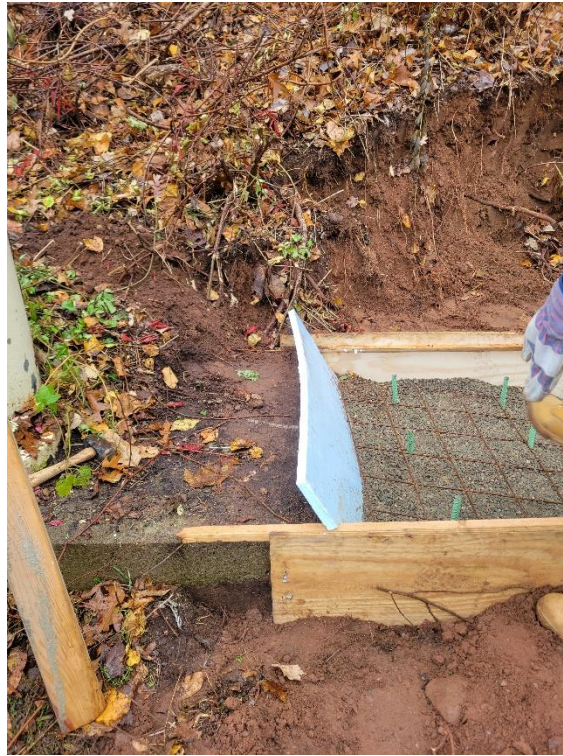
Figure 2.8. Expansion Joint and Reinforcing Steel
