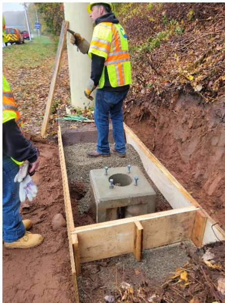
Figure 2.7. Precast Pole Foundation Set to Grade
