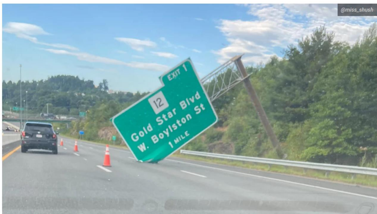
Figure 1.1. Collapsed Sign Support [1]
