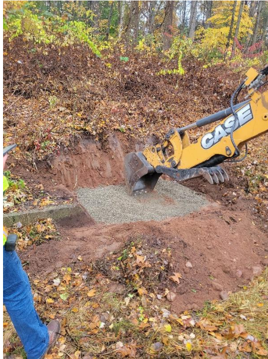
Figure 2.6. Excavation Backfilled with Stone
