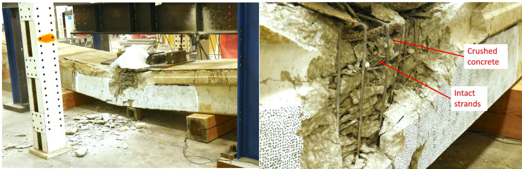
B. Failed specimen
