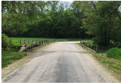
A. View of the single-span bridge
