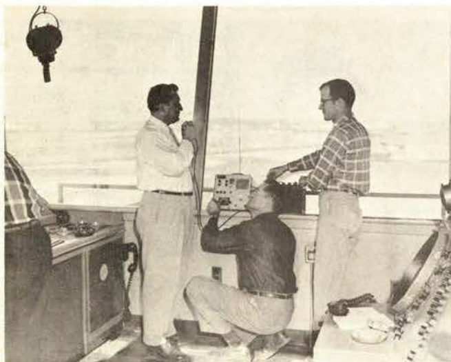
Tower communication following the power failure was re-established by Gonset CAA Communicator providing a portable radio. Seen operating the Gonset unit are (l. to r.) Jim Tate, Air Traffic Communications Specialist; Bob Popejoy, Radar Section Chief, adjusting set; and Robert Elliott, Radar Specialist, holding temporary battery contacts.
