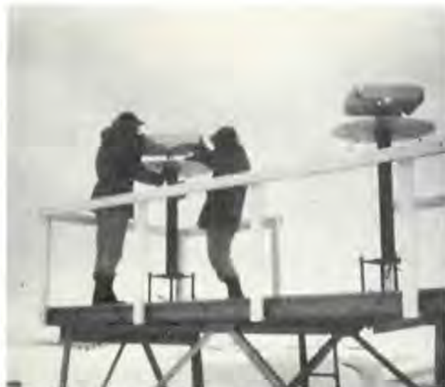
Technicians in Alaska servicing Instrument Landing System Antennas during a heavy snowstorm.
