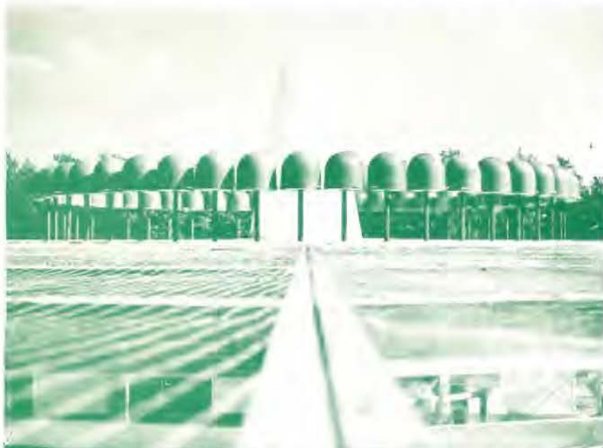
Putting science to work thwarting nature. A 19th century Austrian physicist, Christian Johann Doppler, discovered that sound frequencies coming from a moving source vary in pitch. As applied by the FAA, Dr. Doppler's principle improves VOR (very high frequency omnirange) performance at sites where trees, buildings, wires or other obstructions could interfere with signal reception.
