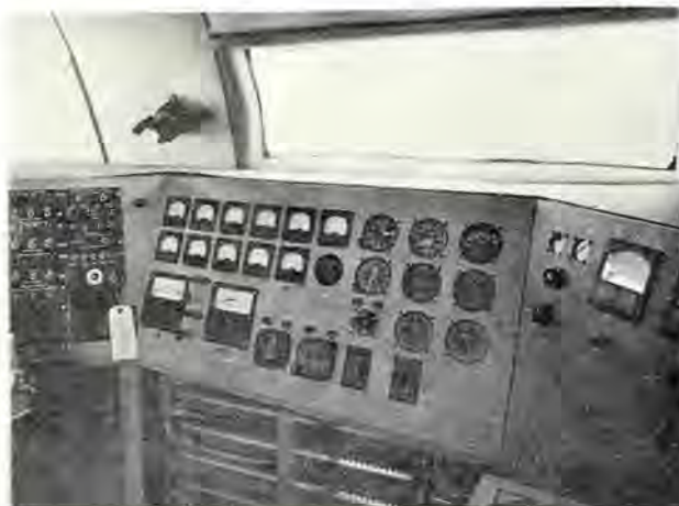
Panel operator's console. Doors are removed to disclose terminal strips and relays.
