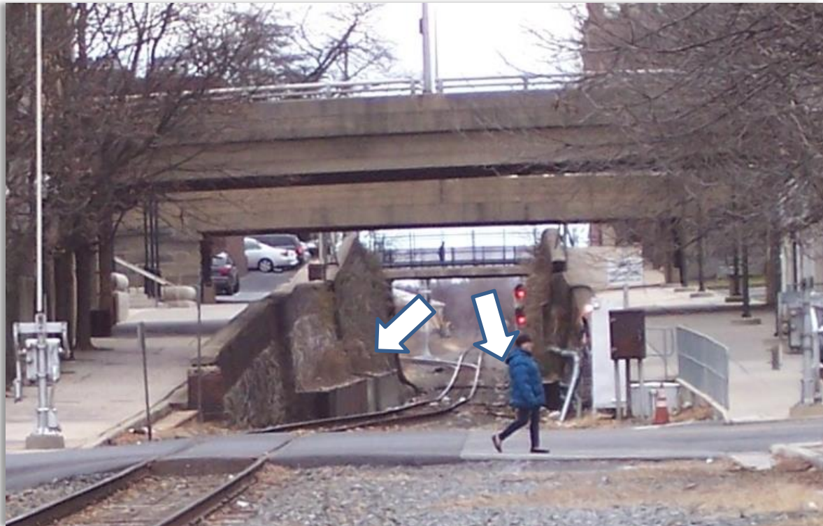
Exhibit 3-35: Concrete Footers on Both Sides of the Reading Cut
