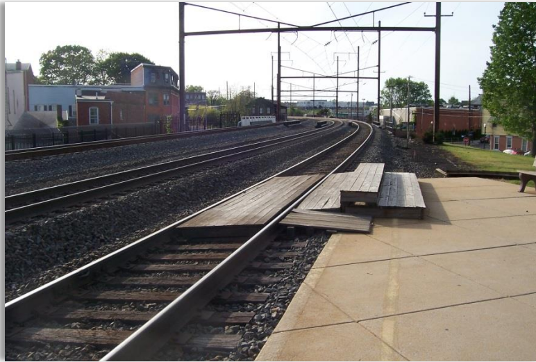
Exhibit 3-31: Wooden Boarding Platform Providing Access to Inner Track
