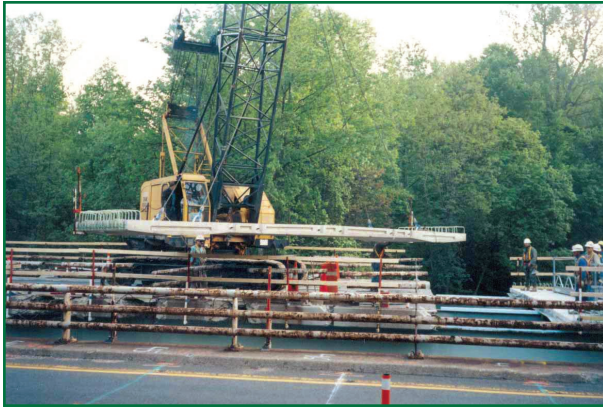
Prefabricated decking enabled repair work on the George Washington Memorial Parkway to be completed on the weekends, when traffic was relatively light.
