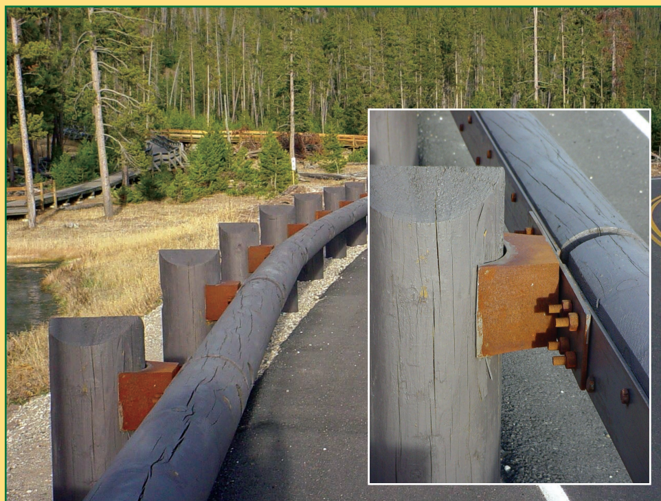
TFHRC supports FLH in developing and crash-testing proposed designs for roadside hardware. A recent collaboration involved steel-backed timber guardrail, shown here installed along a roadway in Yellowstone National Park in Wyoming. Inset: A closeup of the steel-backed timber guardrail.
