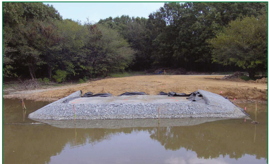
This bridge foundation in Louisiana's Upper Ouachita National Wildlife Refuge employs GRS technology, a solution for soft and frequently wet soils.
