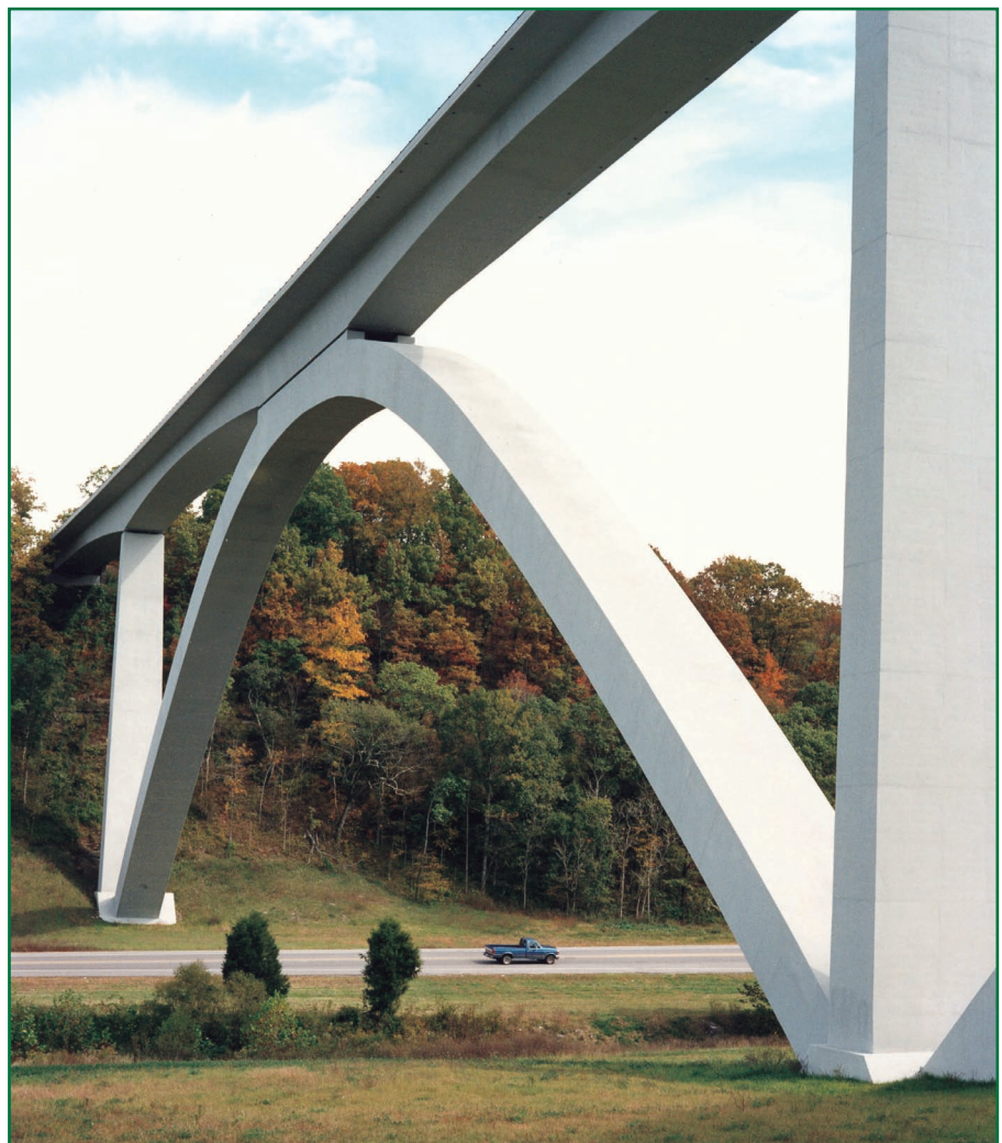
Precasting this segmental arch bridge helped speed construction of the Natchez Trace Parkway in Tennessee.
