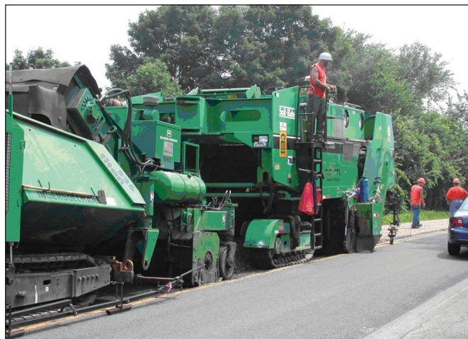
Workers demonstrate cold in-place recycling on a highway project in New York State. FHWA engineers visited the jobsite during a national review of the in-place recycling process.
