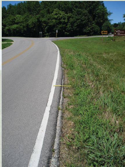
On this two-lane rural road in Stoddard County (left), MoDOT added a paved shoulder, installed edgeline rumble stripes, and placed chevron signs along this curve (right), improving safety for drivers.
