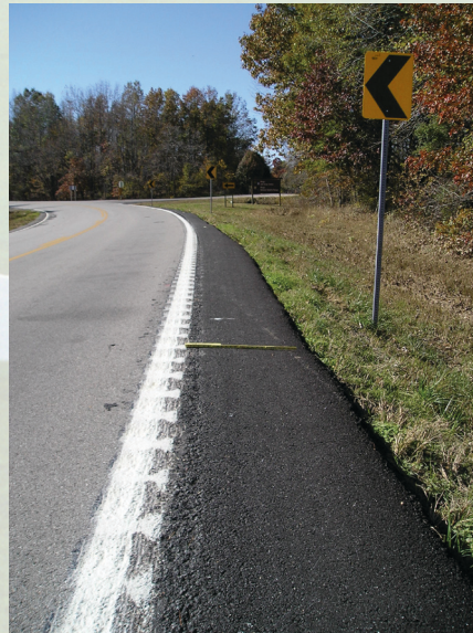
On this two-lane rural road in Stoddard County (left), MoDOT added a paved shoulder, installed edgeline rumble stripes, and placed chevron signs along this curve (right), improving safety for drivers.
