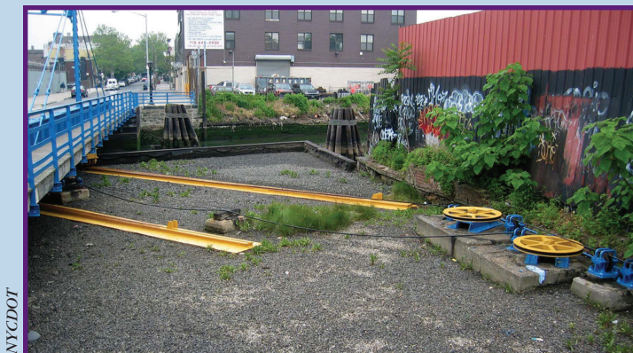
A pair of steel cables attached to pulleys (above, right) pulls the Carroll Street Bridge roadbed (left) away from the Gowanus Canal to enable water traffic to pass without obstruction. The pulley direction is reversed to move the roadbed back into place.
