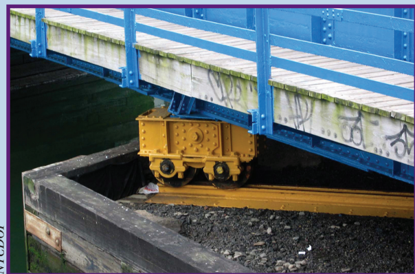
A set of railroad-type wheels under the bridge rolls the structure's roadbed away from the canal to create a clear channel for water traffic.
