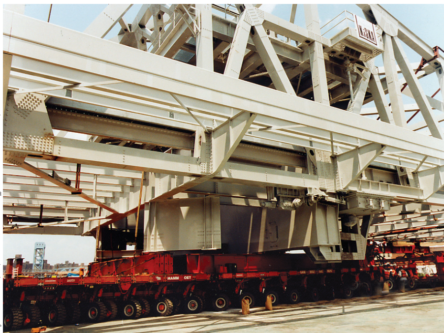
This photo, taken south of the existing Third Avenue Bridge over the Harlem River, shows large, self-propelled transport units used to position the new swing span for transfer to two barges.
