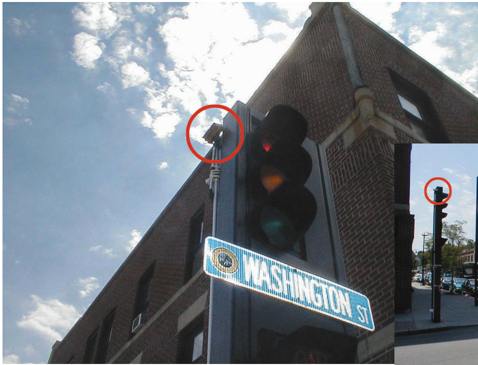
(Right) FHWA researchers installed a stereo camera at this intersection in Norwood, MA. Photo: Migra Systems, Inc.
