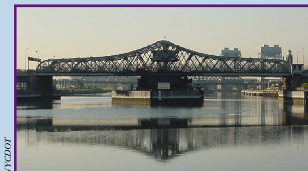
The bridge shown here is an example of a swing span.
