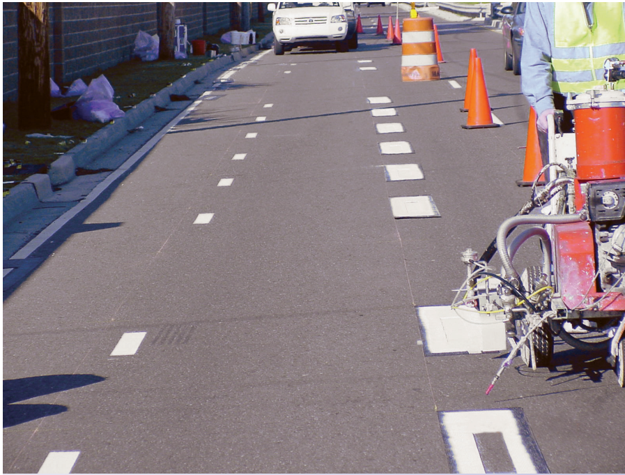
During testing of all-weather pavement markings for work zones, workers used a hand cart to apply paint samples with varying thickness, bead mixture, and other variables to a New Orleans, LA, roadway.
