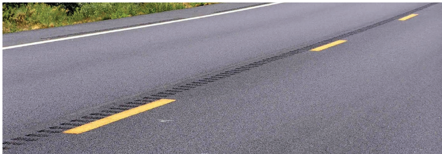
Shown here are milled CLRSSs installed in a two-way passing zone on an Arizona roadway.
