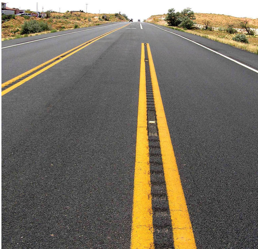
ADOT installed milled CLRSSs at this left-turn pocket.
