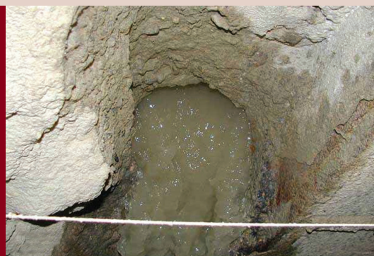
A construction defect in slurry wall panel E0-45 in the I-93 northbound tunnel of the Central Artery/Tunnel Project led to this major water infiltration.
